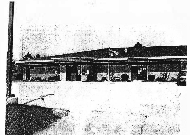
This is the current library. It was built during the early 1990's.
