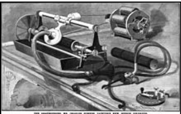
American Graphophone's 1888 wax cylinder graphophone. The machines were marketed for only a few years by American Graphophone and the North American Phonograph Company, but were superseded by Edison's 1888 'perfected phonograph' and its solid wax cylinders.
